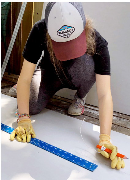
Maddie Rimmer measures drywall to be installed in a Houston home.
